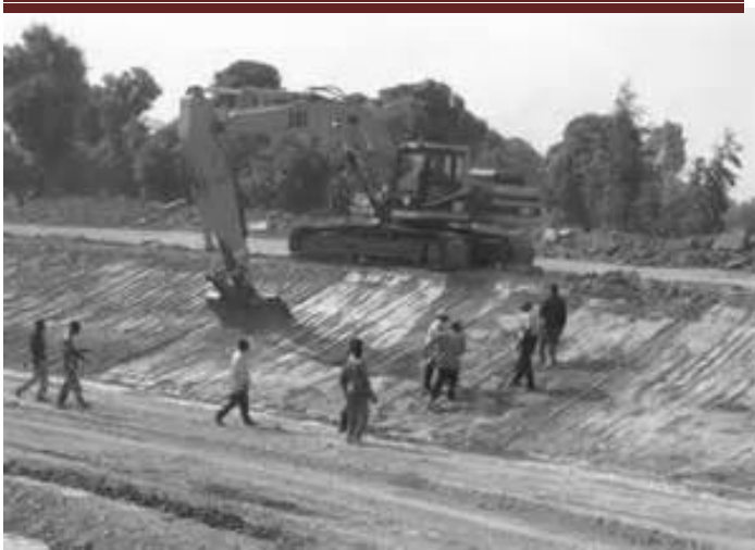
Figure 11: construction de route
